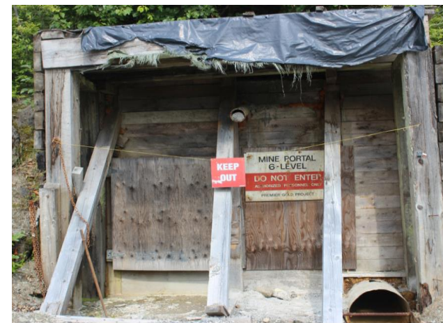
Mine Portal 6 Level
