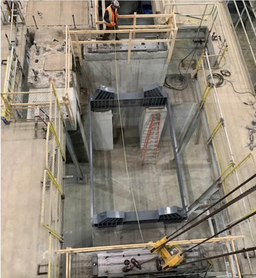
Figure 2 Ball mill cradle being installed.
