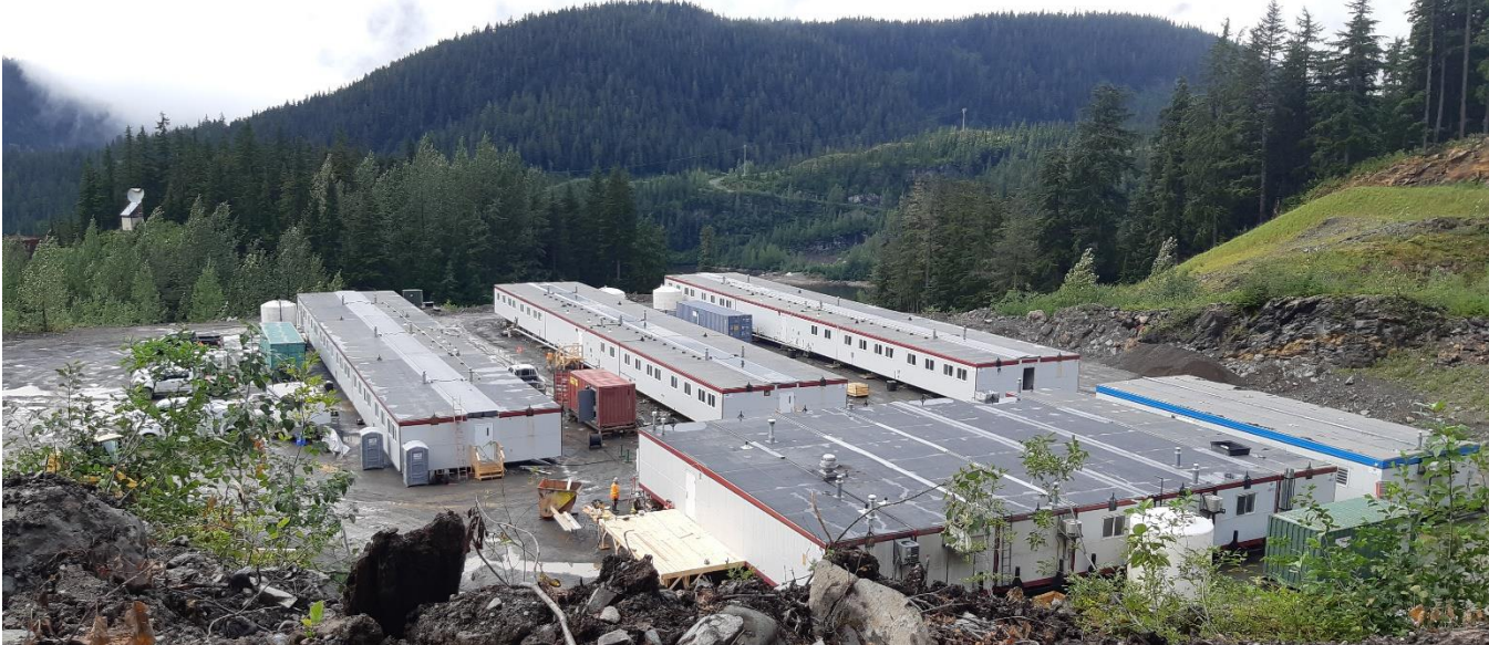
Figure 6 Construction camp progress, 3 out of 4 dorms installed.
