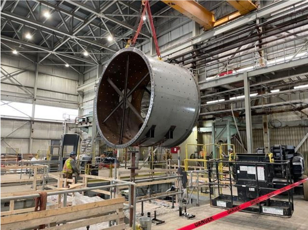
Figure 3 Ball mill shell being lowered into the cradle.
