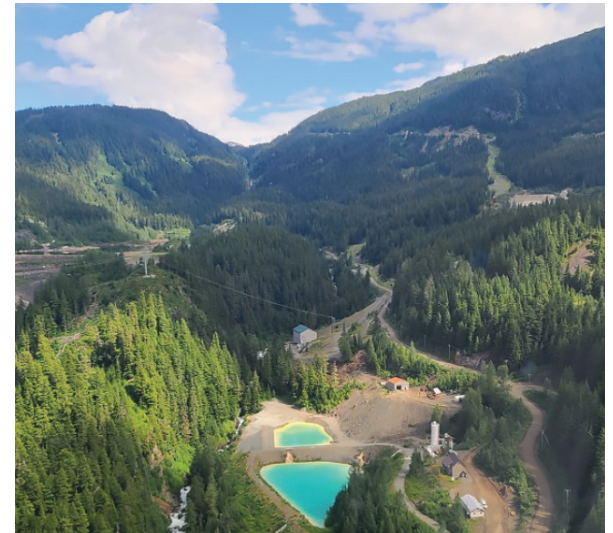
A view of our existing water treatment plant facility that will be upgraded in 2022
