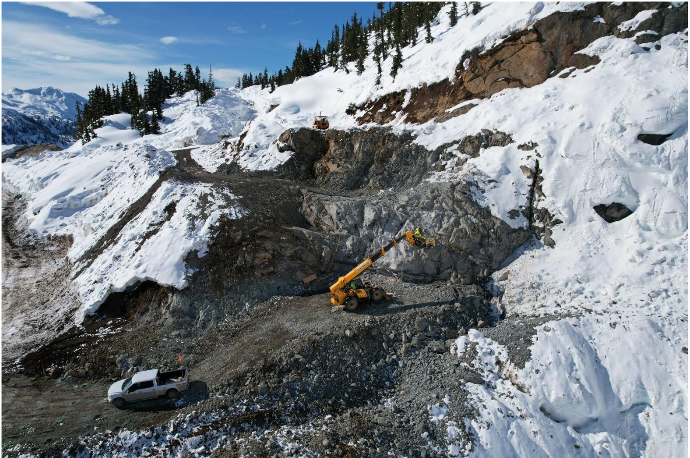
Figure 1 – S1 Portal face being prepared
