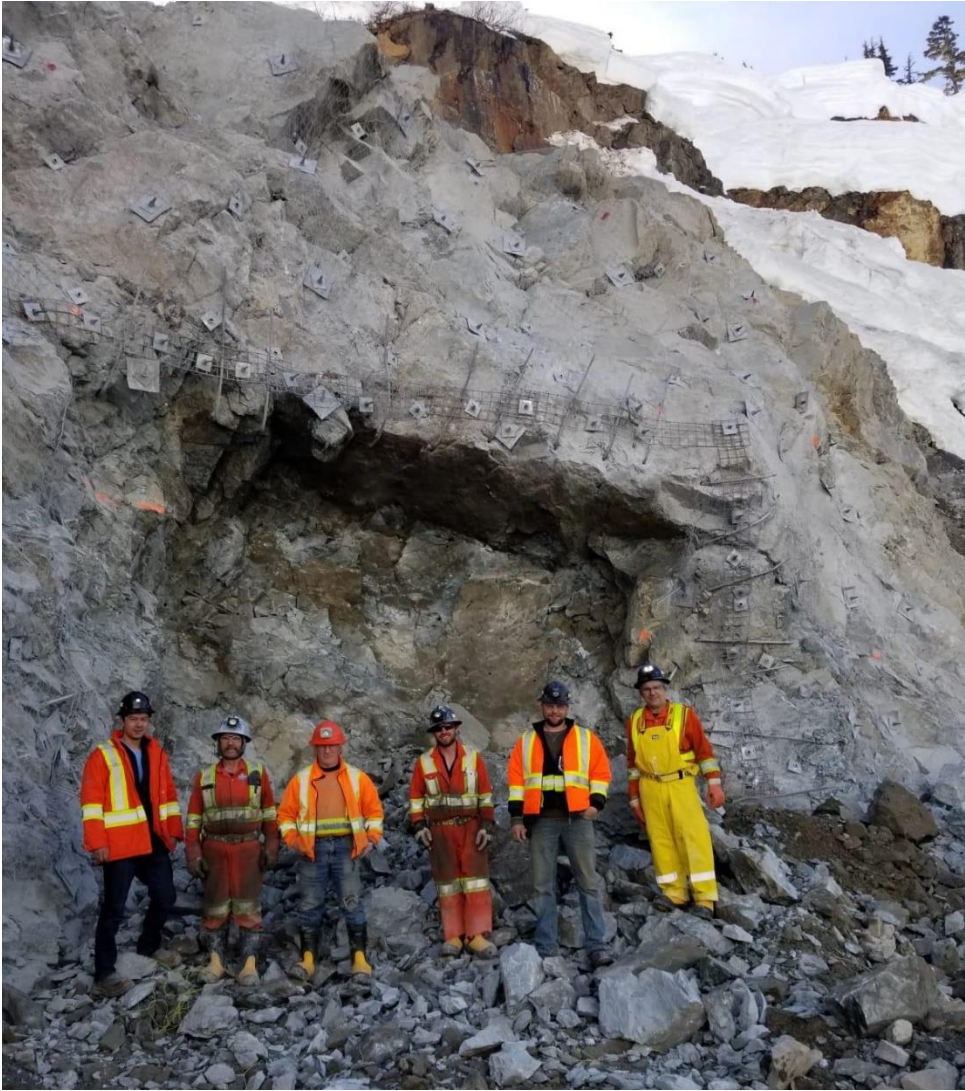
Figure 2 – First portal blast taken
