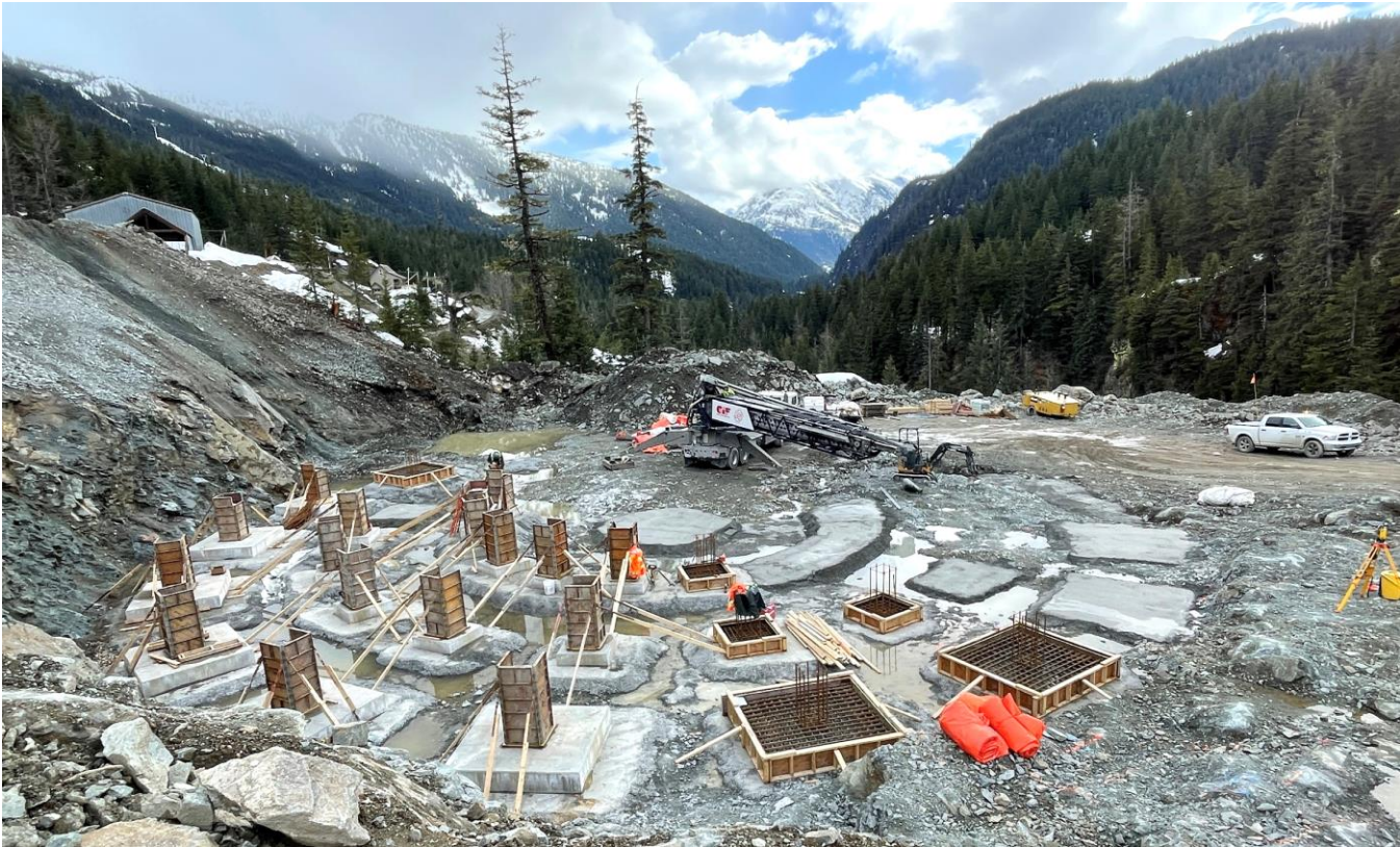
Figure 7 – New clarifier pad foundation construction
