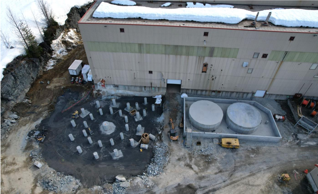
Figure 7 – New clarifier pad foundation construction
