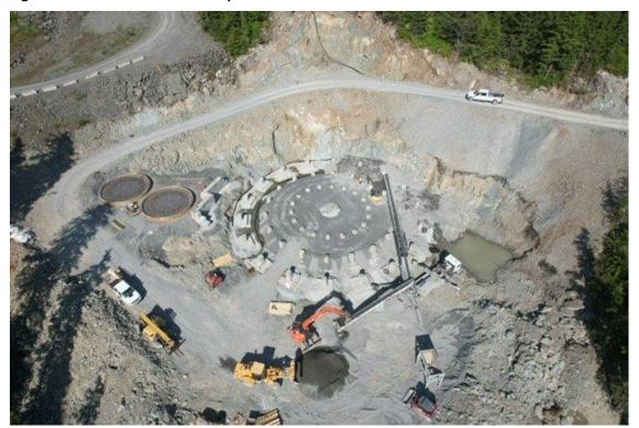
Figure 4 – New water treatment plant clarifier and lime tank foundations
