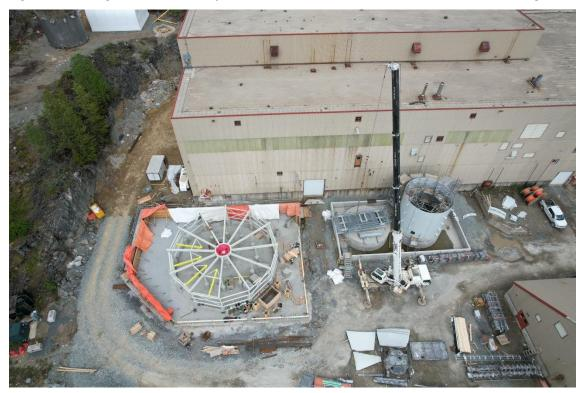
• New water treatment plant: Excavation of the location for the new water treatment plant clarifier was done in 2021. Recently the foundation pad was prepared, and significant progress has been made on the 42-meter clarifier foundation and pedestals. The foundation for the Moving Bed Bio Reactor has also been completed. Work on the new water treatment plant will be placed on hold until alternative financing is arranged, with a
