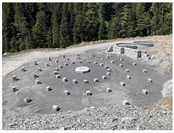
Figure 5 – New water treatment plant clarifier foundation pedestals and lime silo foundations
