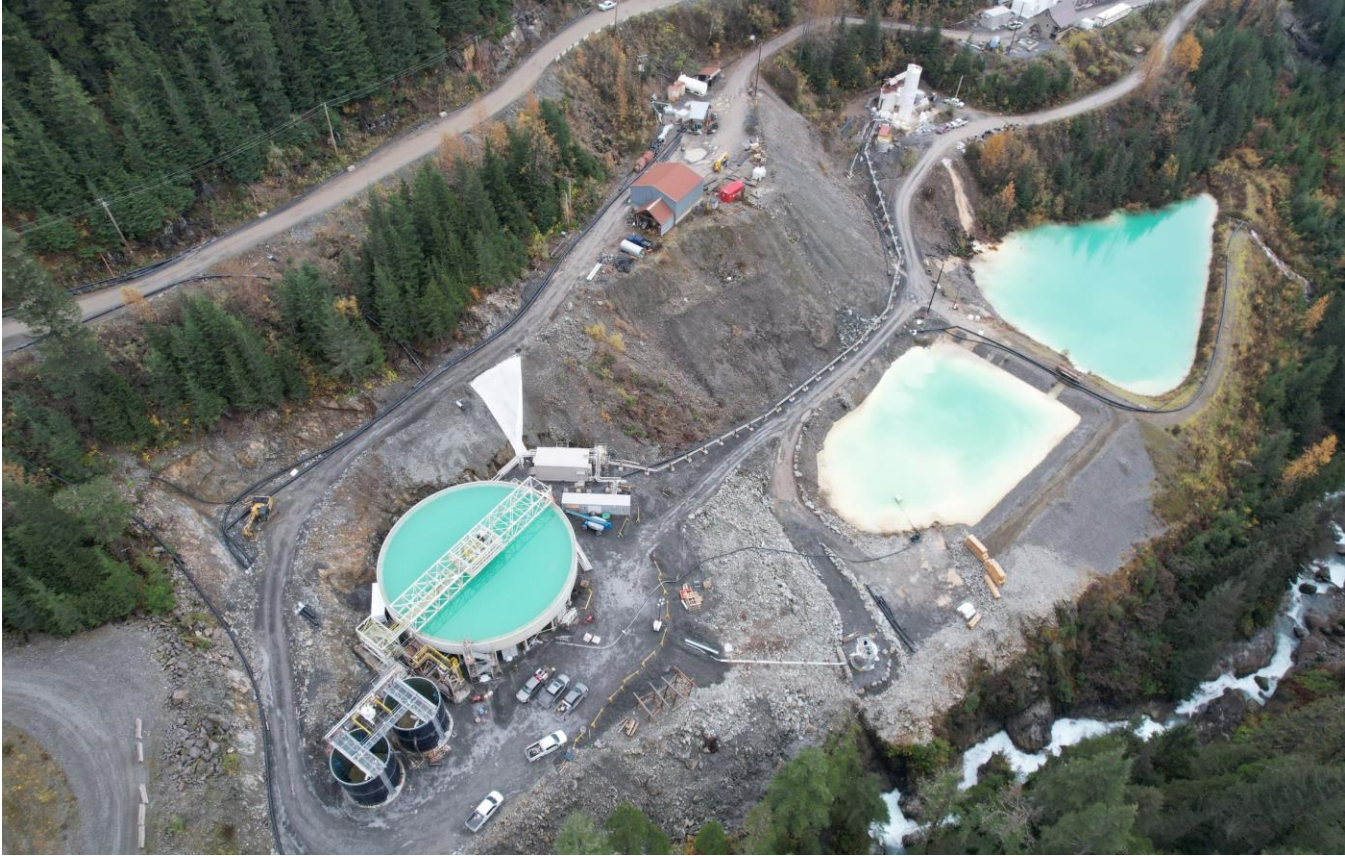
Figure 3 – New WTP overview
