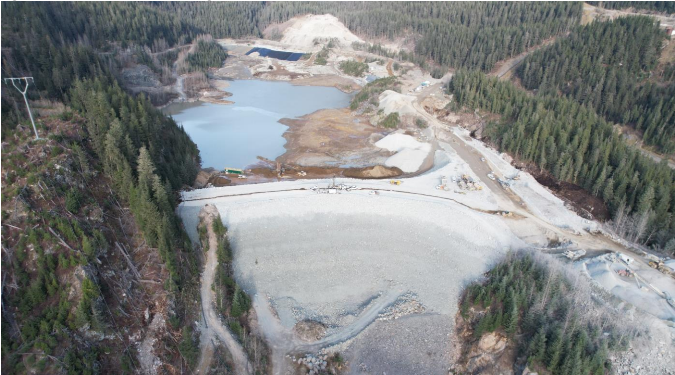
Figure 6 – TSF construction looking north
