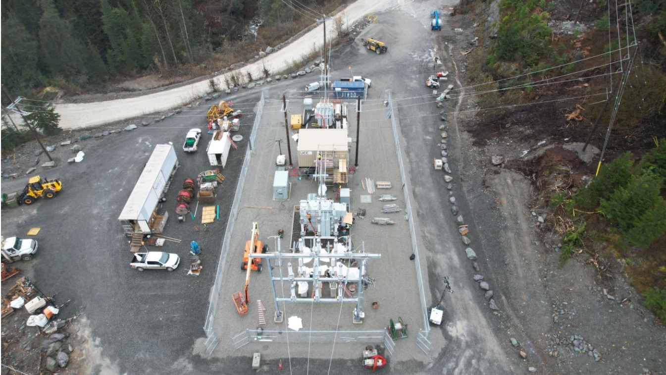
Figure 2 – New electrical substation construction
