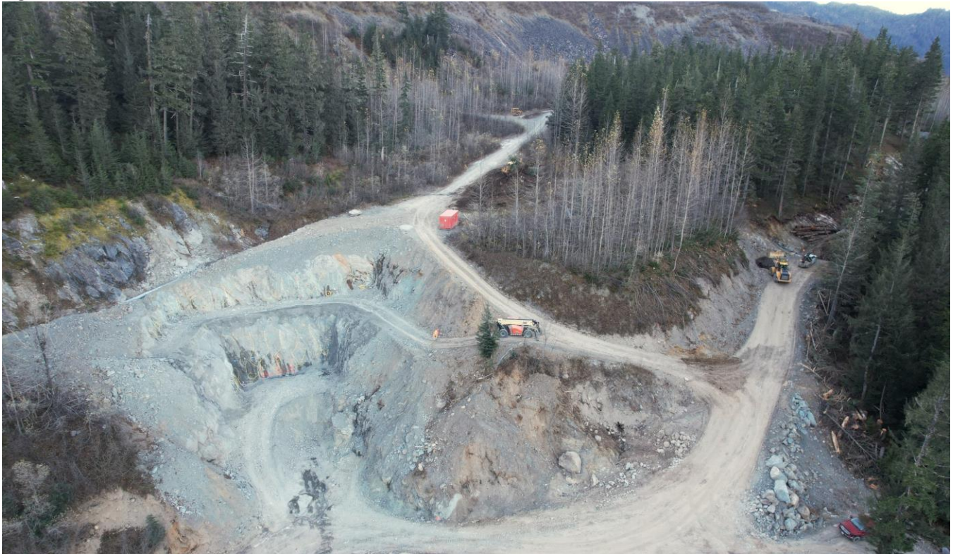
Figure 1 – Premier Portal construction
