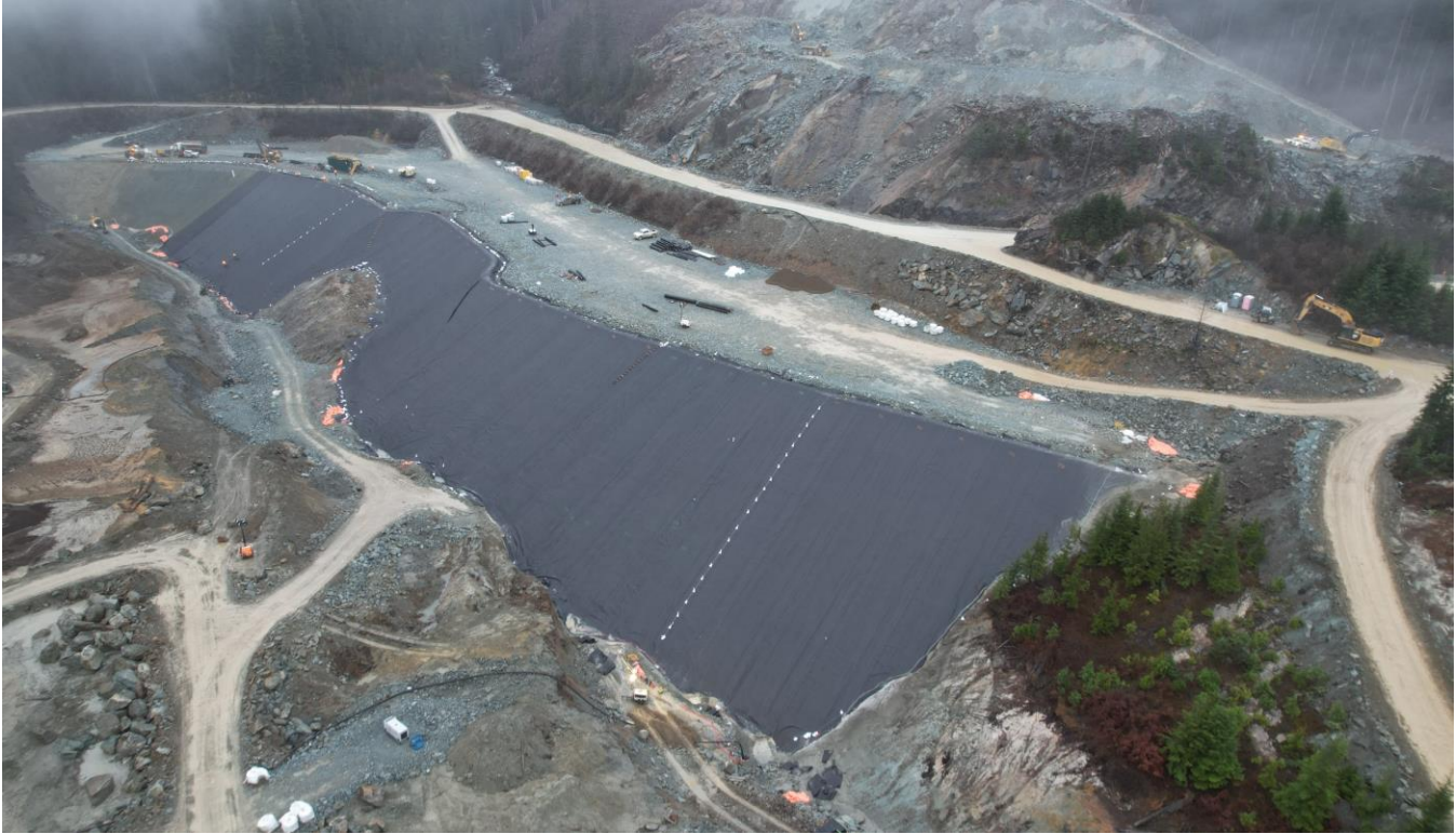
Figure 8 – TSF north dam liner installation
