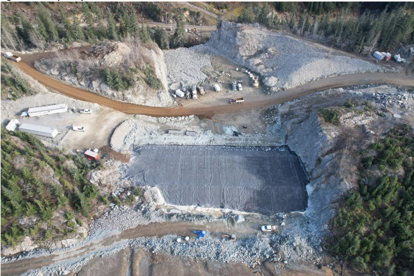
Figure 7 – TSF spillway liner installation
