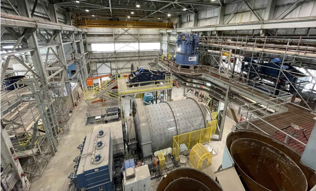
Figure 5 – Process plant interior
