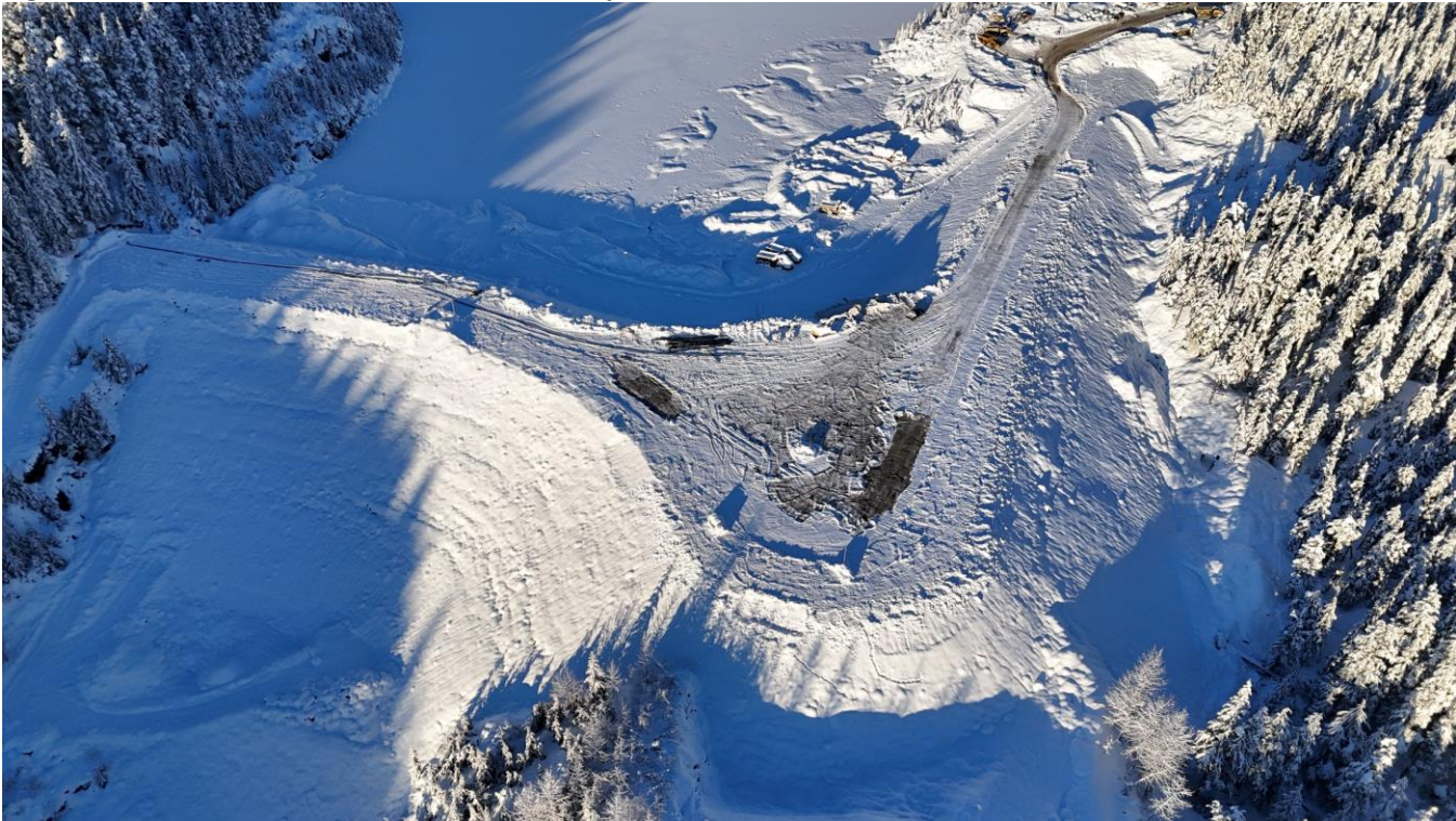
Figure 3 – TSF South and Southeast dams complete
