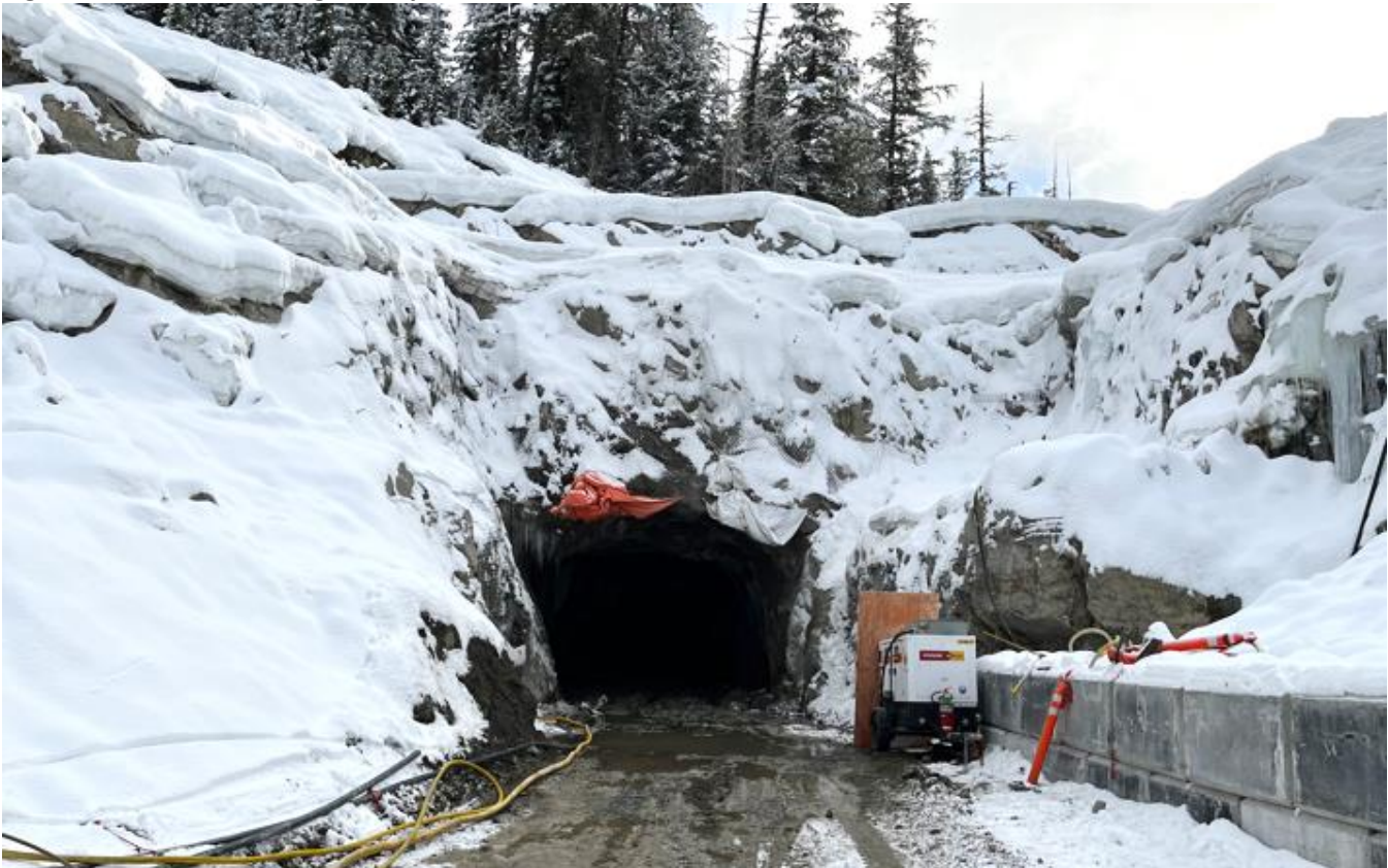
Figure 8 – Premier underground portal front view
