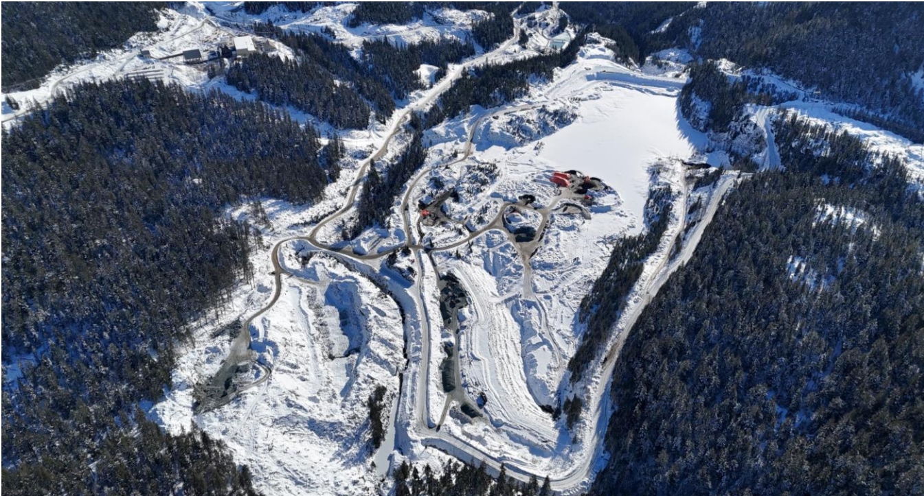
Figure 2 – TSF overview looking south
