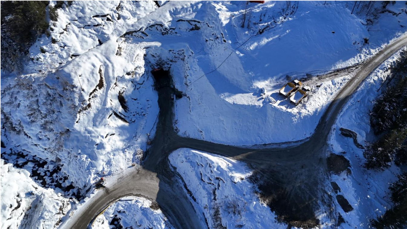
Figure 7 – Premier underground portal overhead
