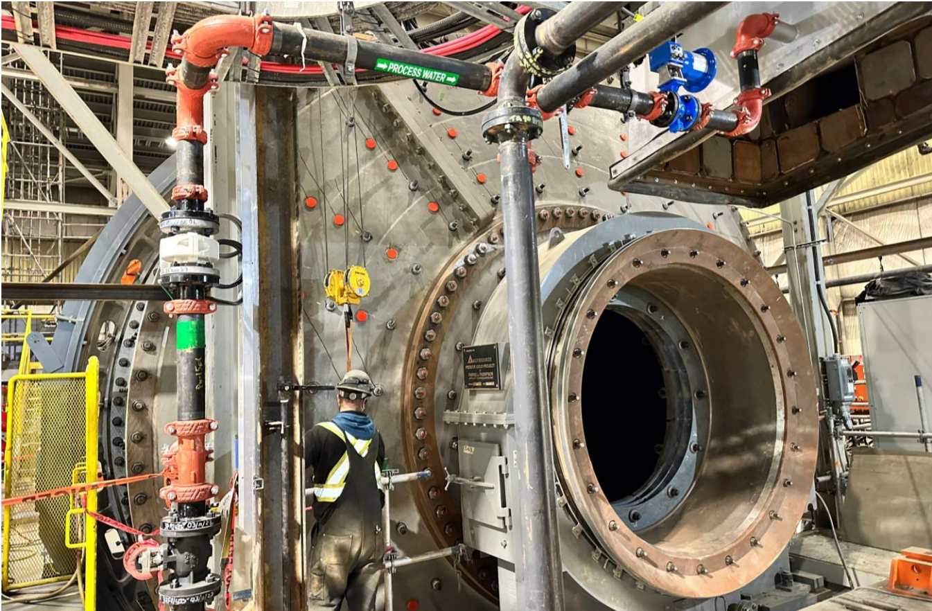
Figure 6 – Mill piping over 90% complete
