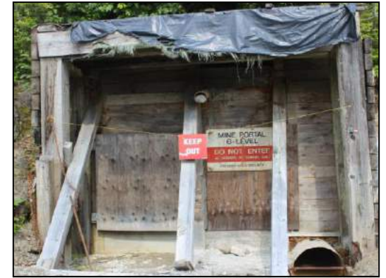
Mine Portal 6 Level
