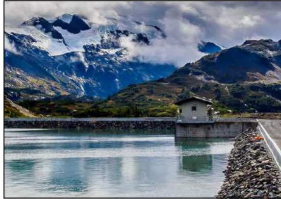
Long Lake Hydro Dam
